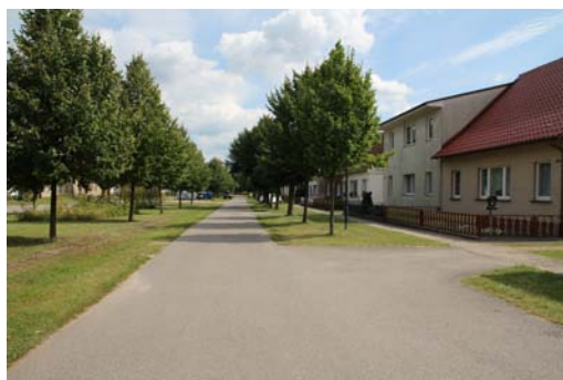
Dorfanger in Meiersberg -Bitumenstraße
